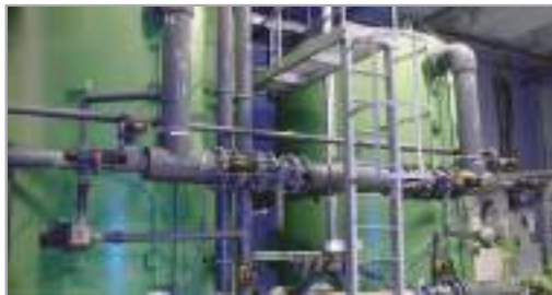
Environmental protection equipment
